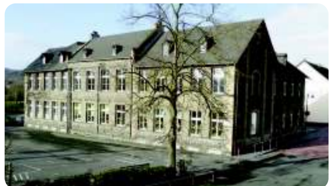
School in Plaidt - Germany
