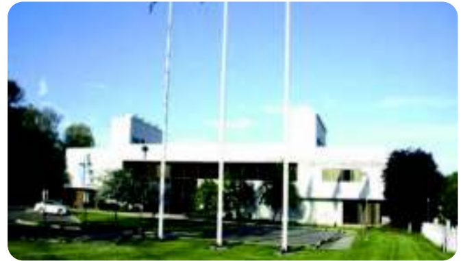
Southern Connecticut Gas Utility - USA
