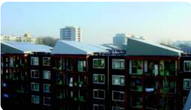
MFH 2 MW Project - Netherlands
